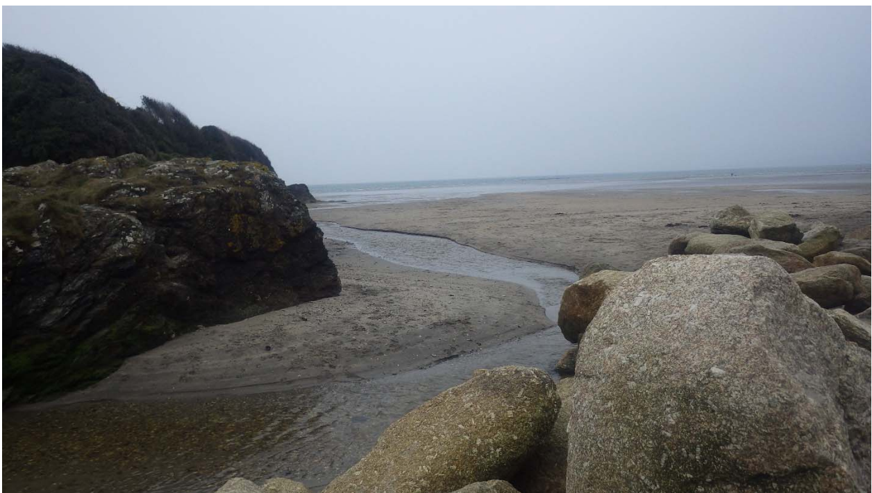
Photograph 2.3 River bank stabilisation placed in 1970s (view seawards)
