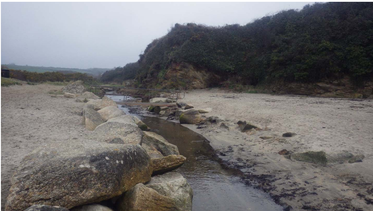
Figure 4.5 Rock boulders in Polmear stream, used to stabilise the channel (taken during site visit 12 th March 2015, above – looking south and below – looking north).
