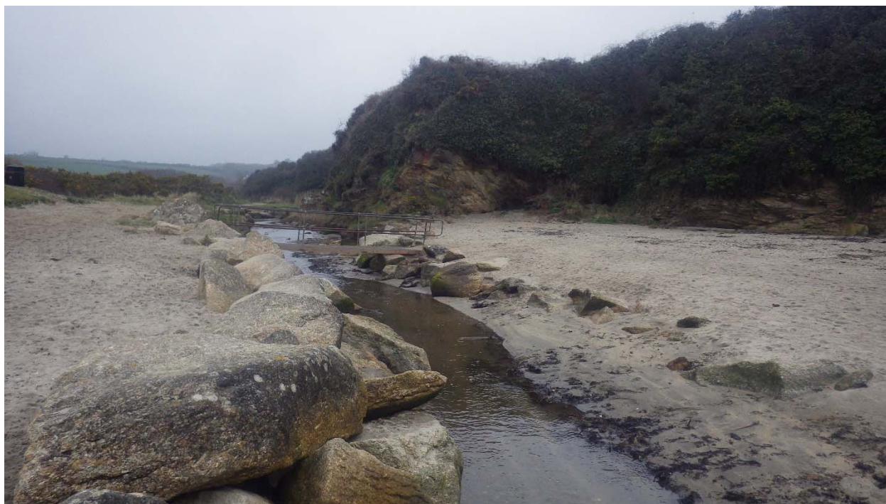
Photograph 2.4 River bank stabilisation placed in 1970s (view landwards)
